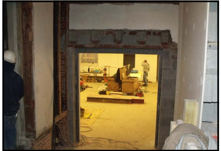
Looking down at the new Fellowship Hall entrance.
